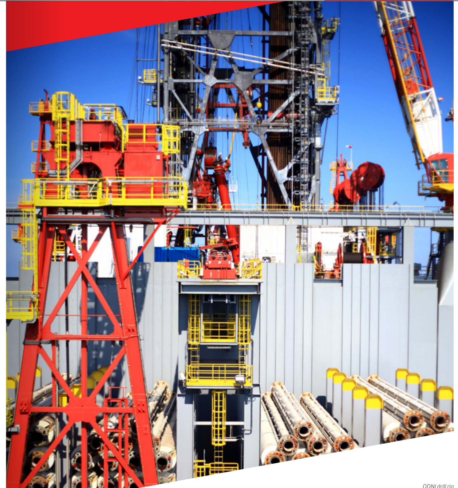
ODNI drill rig
