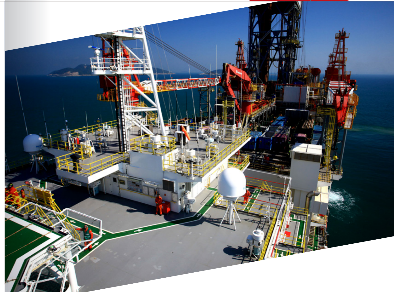
ODNI drill rig
